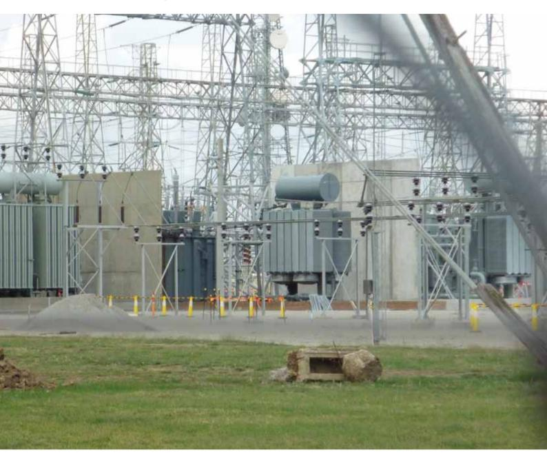
Circuit Breakers (OCBs) when a fault occurred. Both the circuit breaker feeding the fault and the incoming circuit breaker failed to trip. The upstream protection was slow in operating and the circuit breaker feeding the fault exploded, killing both of the electricians in the substation. In the ensuing accident investigation it was found
