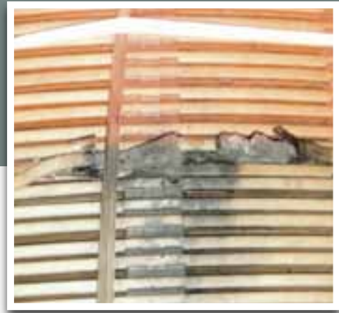
Inter-turn fault, verified by comparison of commissioning winding resistance tests and tests after a fault trip
