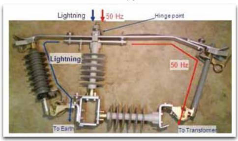
Figure 6: Illustration of the operation of the Combi unit
