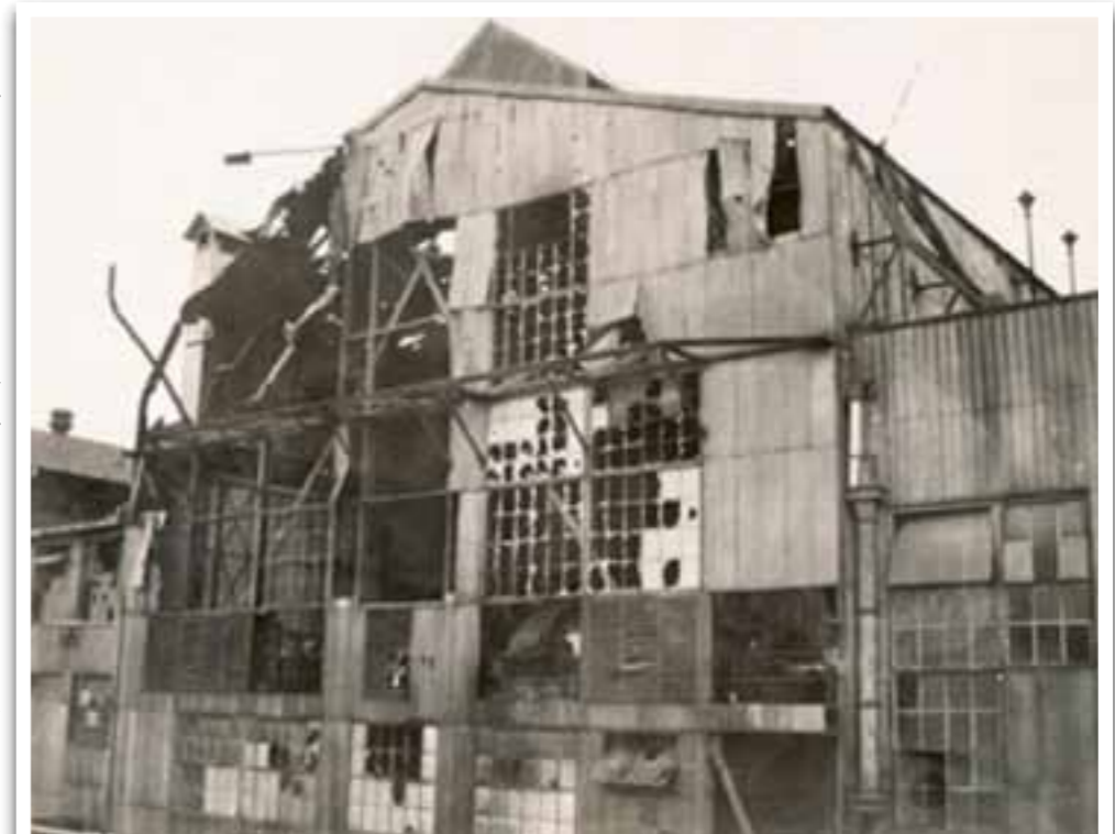
Figure 4: The Outer Wall of the Vereeniging Power Station 1925
