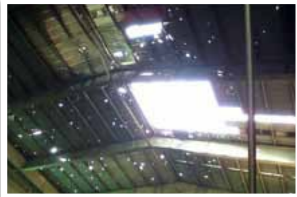
Figure 3: The Roof of the Duhva Turbine Hall
