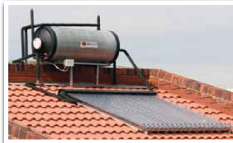
Thermo-Siphoning Solar-Heated System
