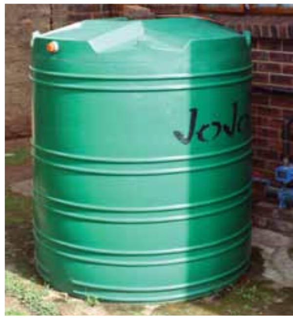
We installed a 2000-litre-JoJo tank.
