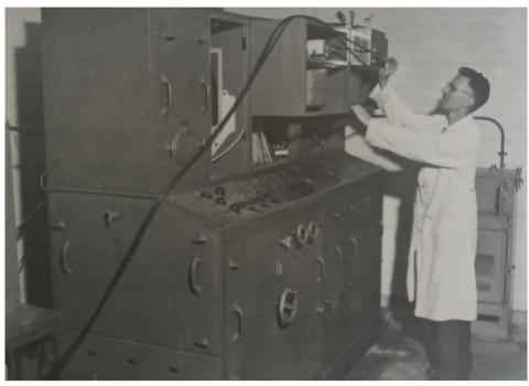
Figure 3: Jules Fejer adjusting the equipment used at the TRL to measure particle reflections, cross modulation and absorption in the ionosphere.
