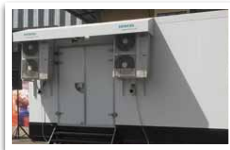
Figure 2 Fully Assembled E-House
