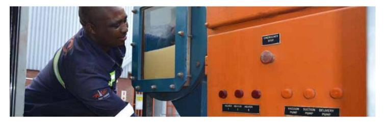
When drawing the oil sample, the sampling technician will also do a visual external inspection of the transformer against a checklist as this will pick up any physical issues with the transformer. Evidence of leaks or a change in colour of the silica gel will be a clear indication that there is moisture ingress. The general condition will also give an indication of corrosion.
