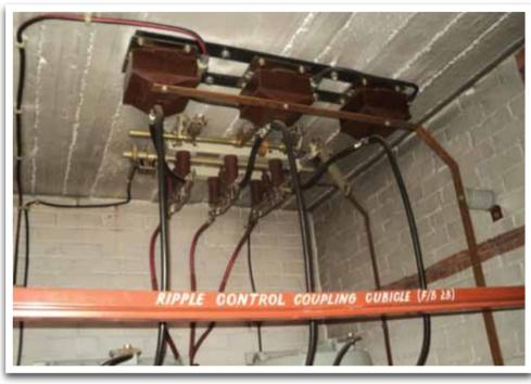
Ripple Control Coupling Cell
