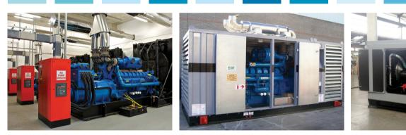
Six 2 000 kVA open type synchronising generator sets Containerised 1 250 kVA generator set
