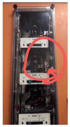
Fig. 9: Operated Protection Relay (Earth Fault Flagged)
