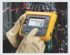
electrical energy waste. These new loggers are easy to set up and use, and capture key measurements - voltage, current, power, power factor, and other variables like temperature - to enable managers to understand their energy usage and correlate it to their activities.
