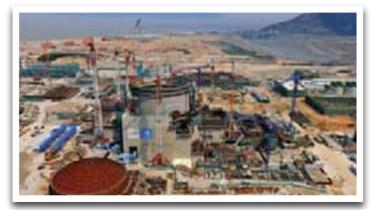
In June, the reactor pressure vessel of Taishan Unit 1 was successfully lowered into place. Source: Areva
