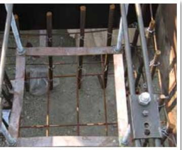
Concealed copper earthing in foundation as applied in Eskom Distribution wattnow | august 2013 | 37
