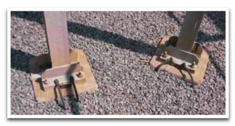
Copper plated steel earth rods used for the earthing of structures in Eskom Distribution
