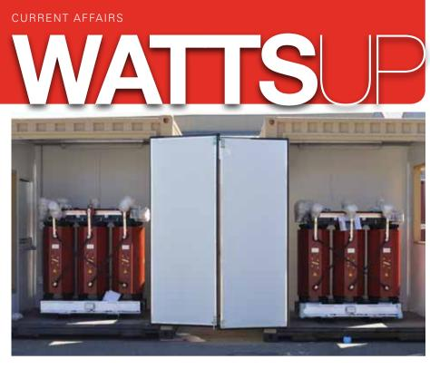
*The Trafo dry-type transformer is ideally suited to this application as it can be mounted inside the modular structure.*
