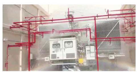
Figure 1: Transformer Sprinkler System
