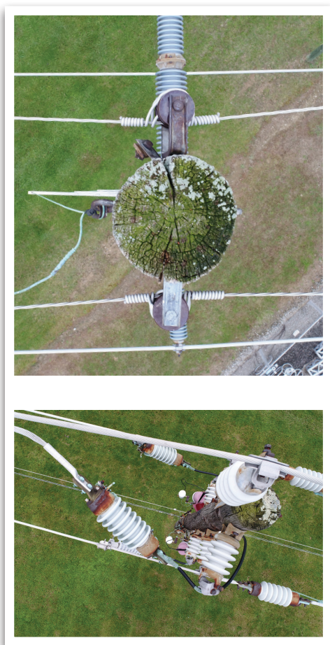
Fig 3 - Inspection Image Examples for Transmission & Distribution
