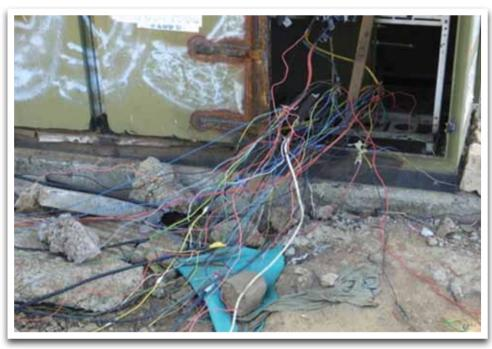
Figure 2: Typical illegal connection from mini-sub.
