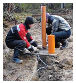
Installation of the level tubes in hard-to-reach locations
