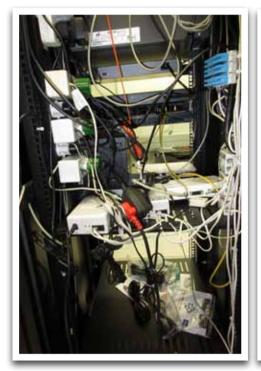
*Figure 3: Showing unacceptable rack wiring.*
