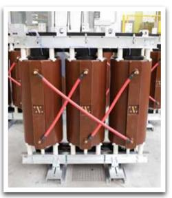
Fig. 3 - Typical cast resin transformer.
