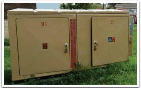
Figure 1: Minisubstation containing 11kV/400V transformer, 11kV ring main unit and low voltage circuit fuses
