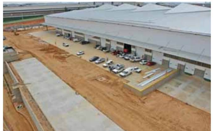
A view of the factory looking across towards Johannesburg.
