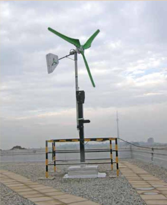
The TechnoSpin wind generator – rated at 2,0 kW at 10 m/s – being commissioned on the roof of the Chamber of Mines building at Wits University.
