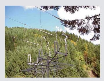
The picture shows what happens when a disconnect switch fails open properly. This was a 115 kV quick break disconnect that had exceeded its switching capability while attempting to de-energize a 40 km section of transmission line Tillamook, Oregon. At times the disconnect switch operated properly, but not this day. As can be seen, one phase successfully disconnected, but the other two phases did not. Luckily the operator was able to reclose the disconnect before it relayed out.
