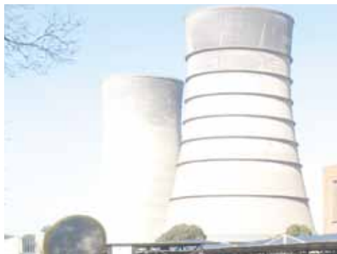
16 July: Tour of Kelvin Power Station. It was interesting to inspect the old generators but disappointing that the machines were not running due to maintenance work.
