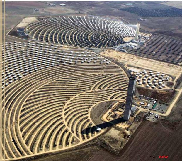
Abengoa's CSP facilities near Seville, Spain. The larger addition (foreground) is called PS20 and is currently the largest in the world with a capacity of 20 MW.
