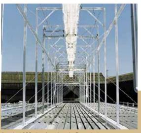
A typical CSP plant based on the Fresnel mirror.
