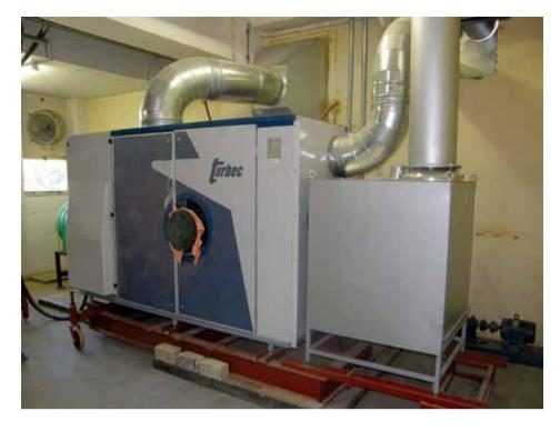
A Turbec 100 kW gas turbine installed at the CSIR as the starting point of the Forty Towns Project. The intention is to drive the turbine using air heated to 800°C by a CSP plant and methane, recovered using anaerobic digestion of sewage sludge.
