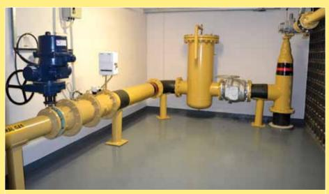
Incoming gas is at very low pressure, which makes it an extremely safe transporting mechanism. The main gas valve is held open against a spring and will shut-off automatically as soon as any sensor detects a leak.
