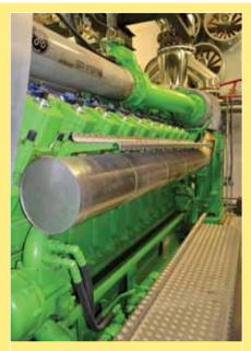
One of the four J 620s from GE installed at the Absa energy centre in Johannesburg. These 20 cylinder reciprocating gas engines have a peak generation capacity of 2,8MW each and emit 40% less greenhouse gases than coal-based generation, making them one of the cleanest combustion based technologies available.
