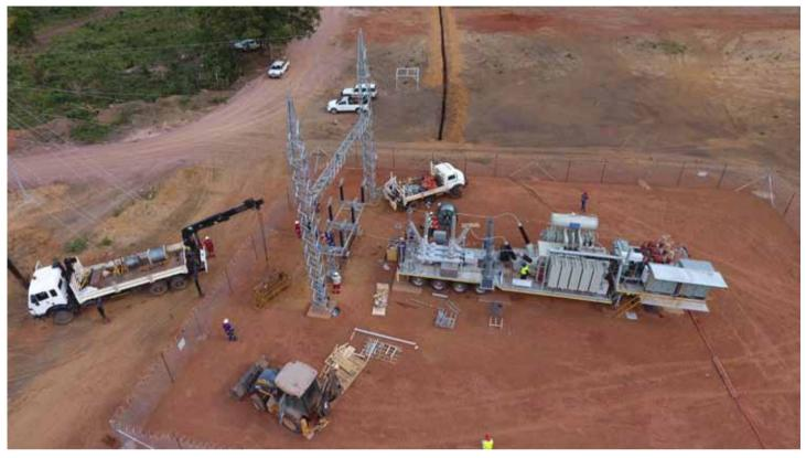
*The Zest Energy mobile substation in position on site, connected to the SNEL electrical network. The photograph shows preparations for hot commissioning and energising in progress.*
