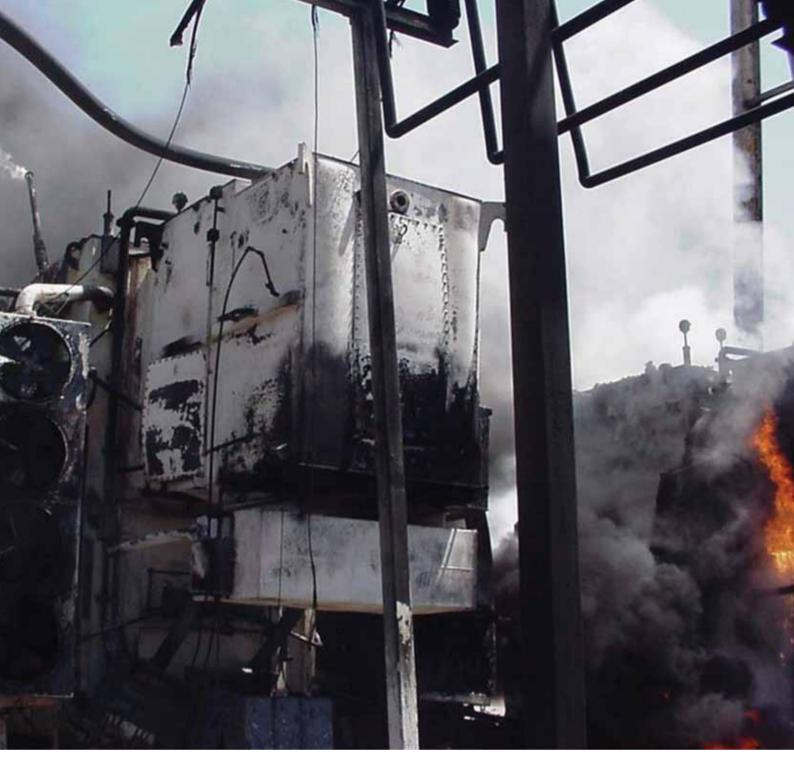
of deterioration that, if ignored, would lead to an internal fault occurring. On one hand, there are fairly accurate guidelines, tolerances and limits in analysing the data of the chromatogram of oil-dissolved gases in determining the condition of the power transformers and the consequent ability to identify faults or problems while still in the incipient phases of development. Furthermore, finding linkages, trend analysis and patterns between DGA and electrical network condition or
