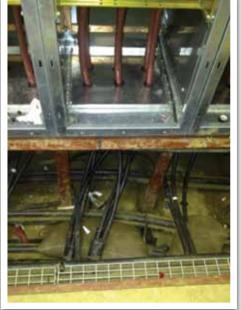
*Example of tri-furcating termination into compact MV switchgear*
