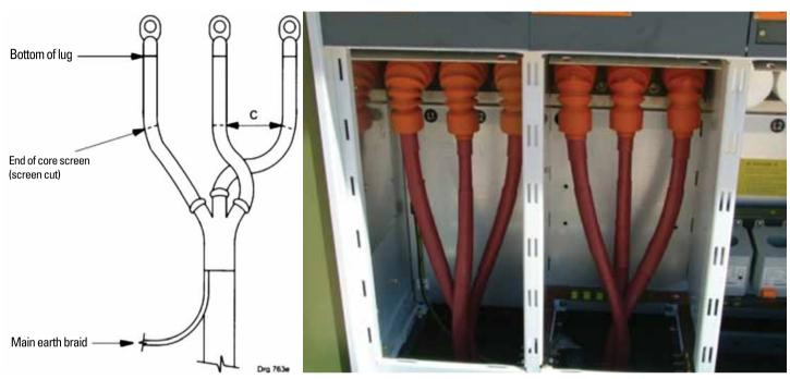
Figure 9: Example of a cable termination where the core crossing is made below the end of the core screen
