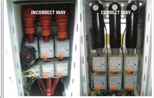
Example of incorrect and correct termination into compact MV switchgear with LV CTs
