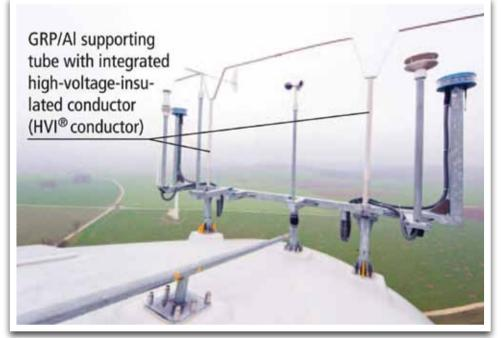
*Figure 2 - Example of an air-termination system for the weather station (anemometer) and the aircraft warning light*
