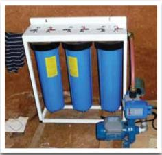
Fig 9. The water filter system.
