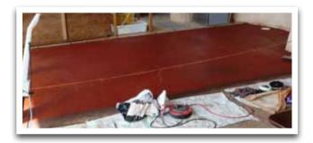
Fig 3. The completed earthen dining room floor.
