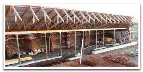
Fig 6. The thermal mass in the southern earthbag wall and the white insulation underneath the metal roof.
