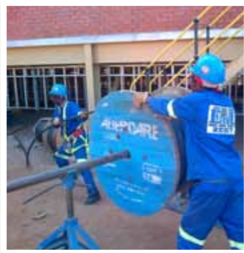
EnI Electrical cable pulling team in Zambia.
