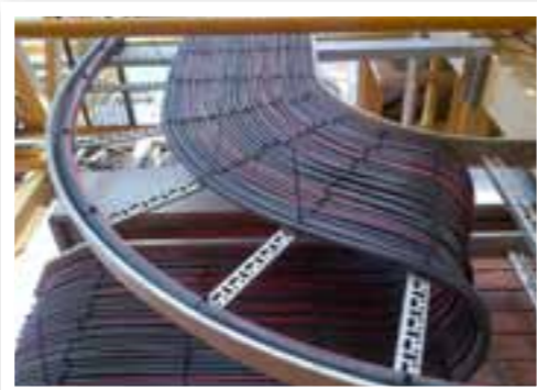
Cable racking done by EnI Electrical in Zambia.
