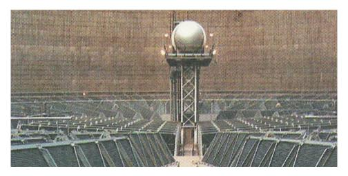
The inside of a Kendal cooling tower, showing some of the hundreds of air-cooled radiators
