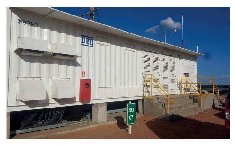
The WEG ESW 750 centralised inverter station, housed in a 12 metre container installed on site.
