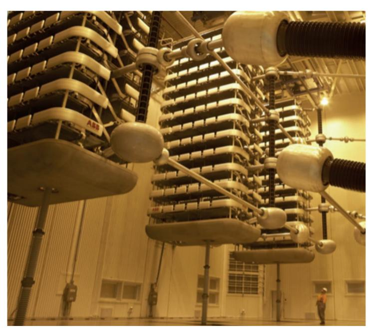
Suspended twelve-pulse ABB thyristors in the valve hall at Haywards in the New Zealand HVDC Inter-Island scheme (The two transformer bushings can be seen on the right)
