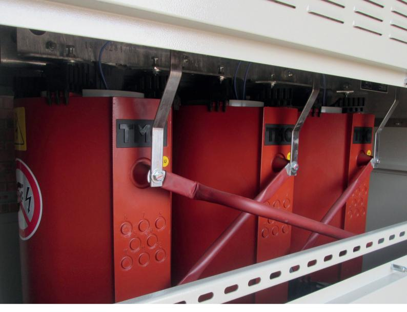
A 400V/22kV step-up transformer designed for renewable energy applications.
