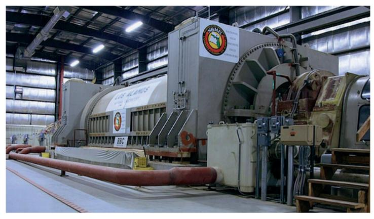
The 1,2 GW motor generator system which powers the outer coils on the LANL 100 T pulsed magnet.
