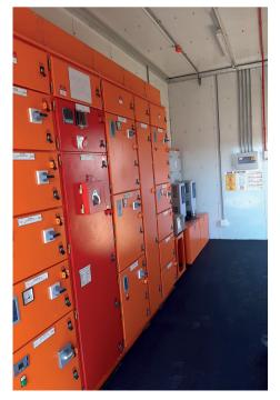
The low voltage (LV) room of the E-House with the internally arc type-tested IEC 61641 MCC.
