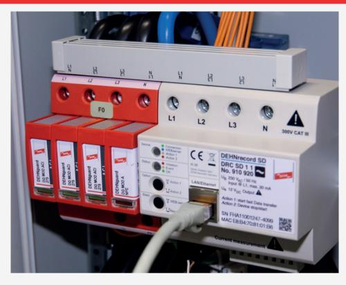
Figure 2: Example of a smart PQ Measurement Device capable of measuring Surge and Lightning Impulse
