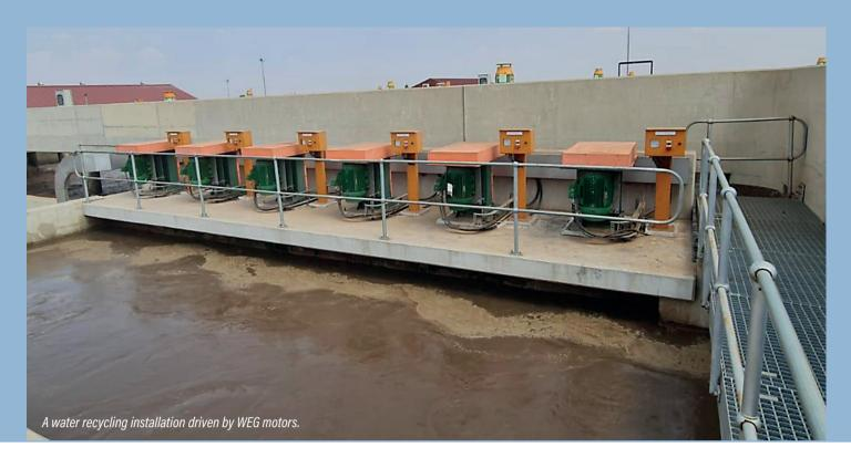
contract also specified including anti-condensation heaters for all motors of 4 kW and above. Our motors on-site also boast paint plan 212P and IP66 ingress protection to help keep them free of moisture or dust."
