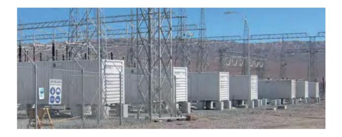
**Figure 3-3 | Li-ion battery supplying up to 12 MW of power at Los Andes substation in Chile** (*A123, 2009*)
