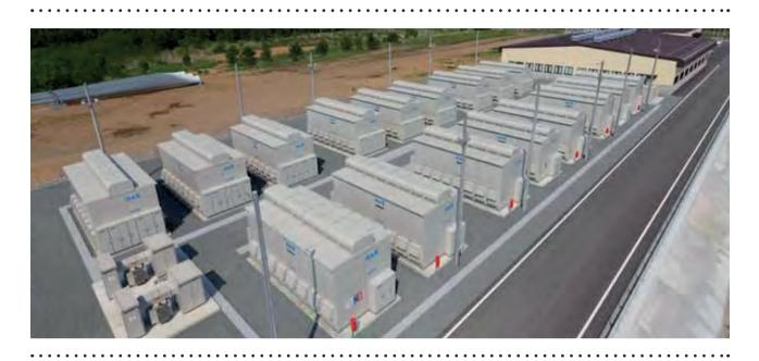
Figure 3-10 | NaS battery units - 34 MW (Japan Wind Development Co.)
