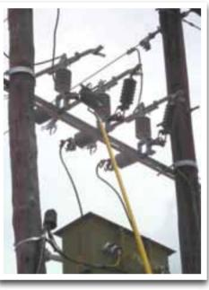
*Fig.8 The live line surge arrestor in the* Combi unit is positioned not further than 1 meter from the transformer, Eskom specification, D-DT-1877.
