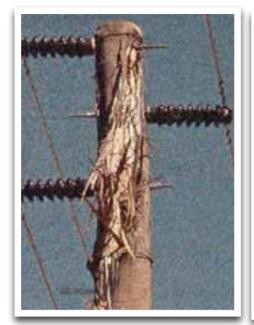
Fig. 7 Lightning damage to a overhead pole, *due to theft of bonding cables to the earth* point.
