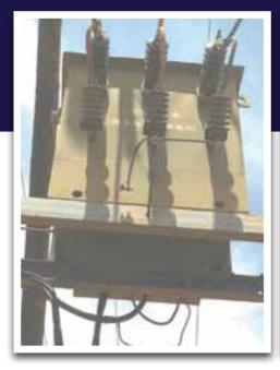
Fig.4 A spent 11kv surge arrestor, that has blown its GLD with no replacement installed. Research reveals this shortcoming is a major contributor to transformer failure rates within Southern Africa, as surge arrestors are not replaced for lengthy periods of time.
