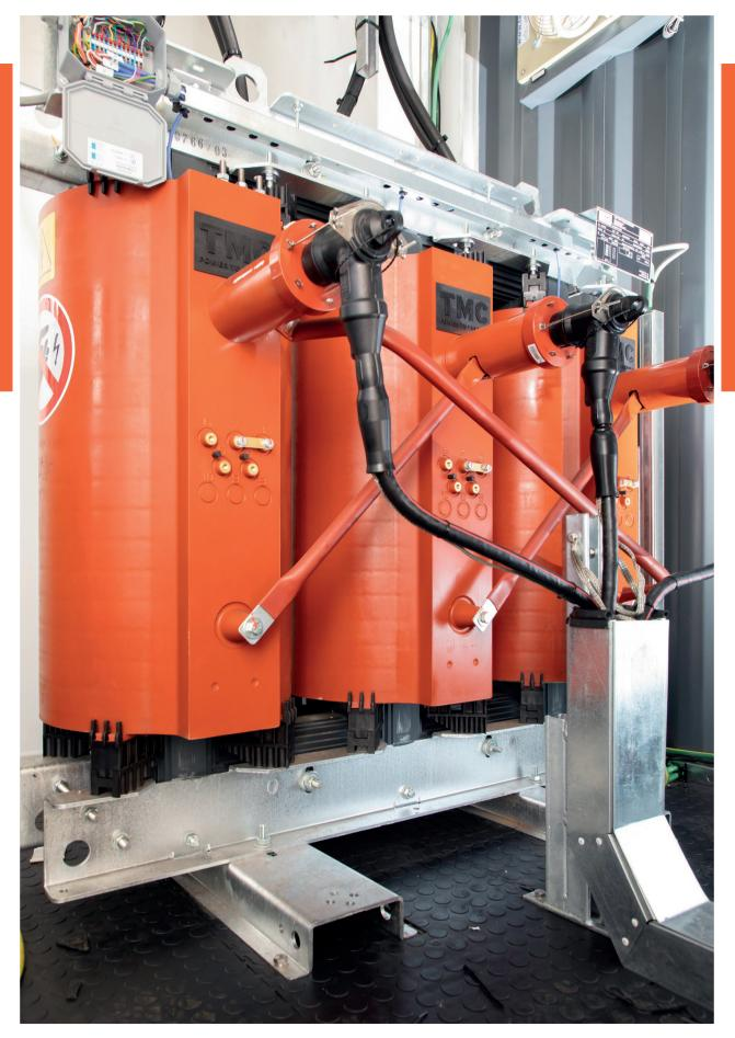
1250kVA cast resin transformer installed inside modular substation.
