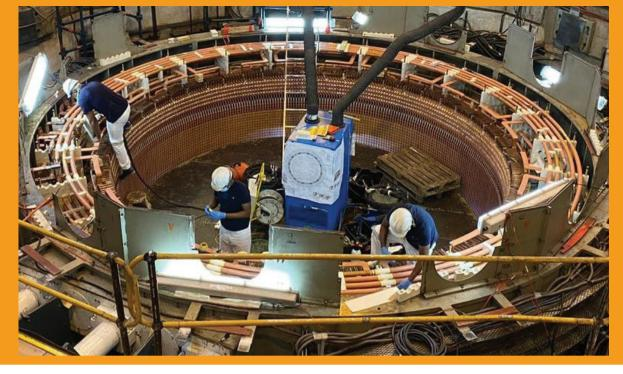
M&C technicians are seen working in the large area left inside the stator after removal of the rotor as they install some of several hundred stator bars as part of the complex stator winding operation.
