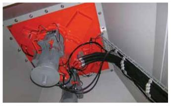
Antenna motor, gearbox, RF and power cables.
