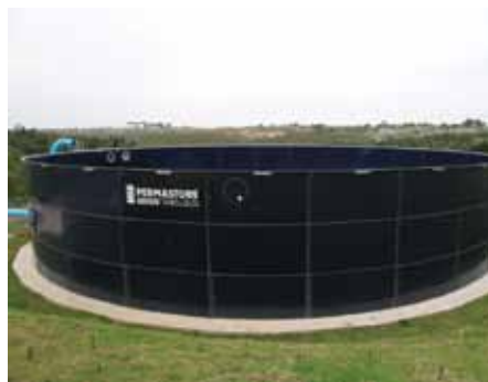
Storage tanks – ceramic coated steel panels.
