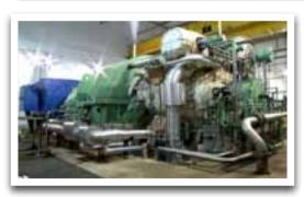
A TGM condensing extraction steam turbo generator set operating at a paper mill in Brazil. This set is similar to that which will be supplied and installed at Mondi Richard's Bay facility.
