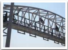
Figure 5. Equipment mounted on open road toll gantry.
