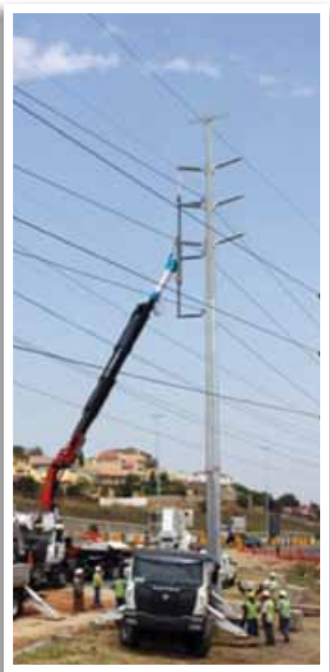
New tower being installed while conductors are still energized
