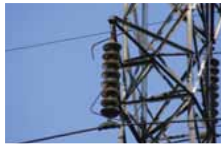
Old porcelain insulators that were replaced with composite silicon insulators
