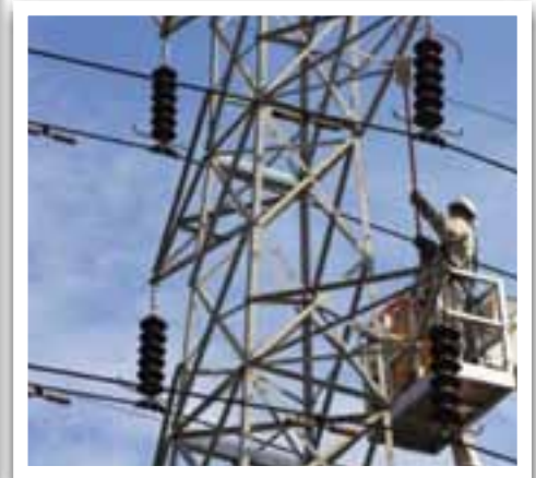
Hotstick technique being utilized to test insulators prior to approach
