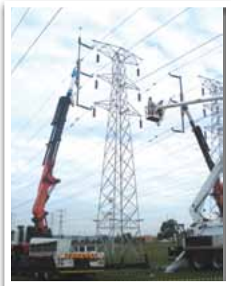
LineMaster robotic arm being utilized to hold and manoeuvre live conductors
