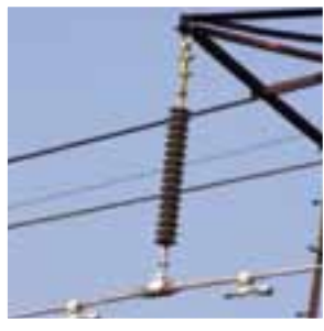
Old porcelain insulators that were replaced with composite silicon insulators
