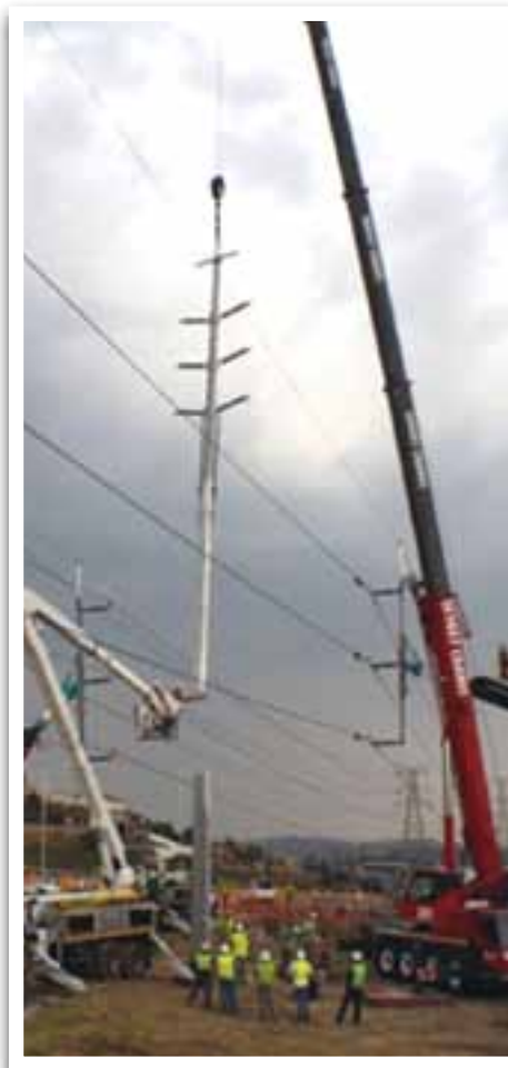
New tower being installed while conductors are still energized
