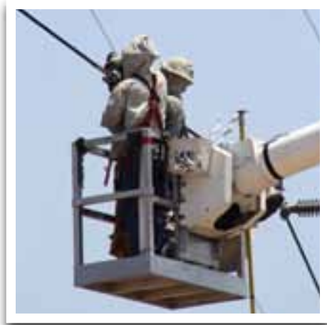
Barehand technique being utilized to install line dampers
