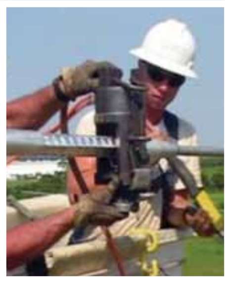
Dead end wedge crimp connectors
