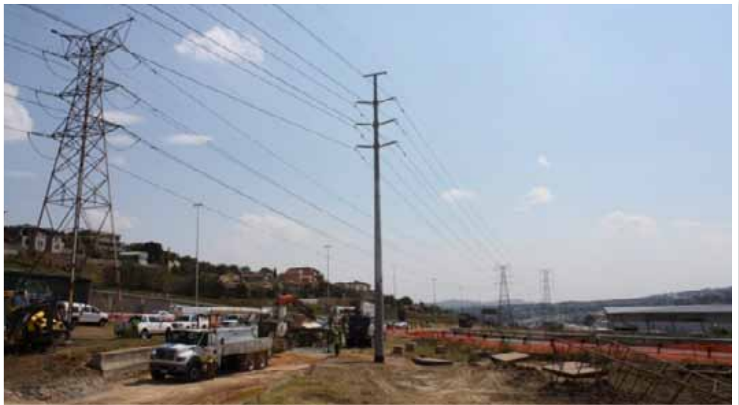
New tower in position with no supply interruptions experienced
