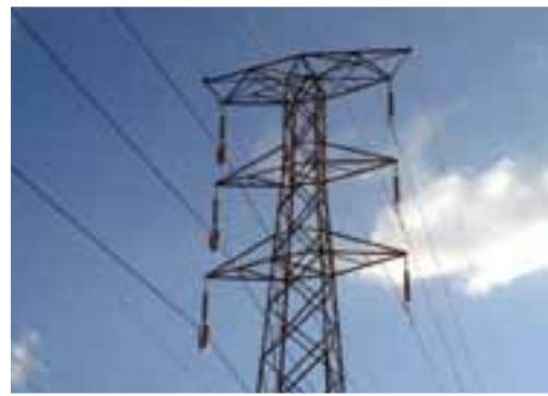
New ACCC conductor being pulled in with old conductor
