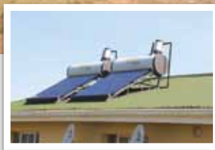
Solar Geyser Installation
